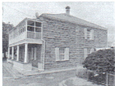
A house in Rudd Lane Oudtshoorn
